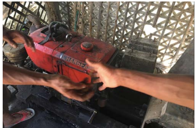
Diesel Generator in Kya Pin
